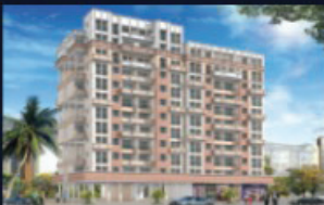
Shelter Residency, Kharghar
