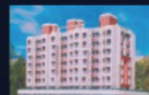
Shelter Complex, Kharghar
